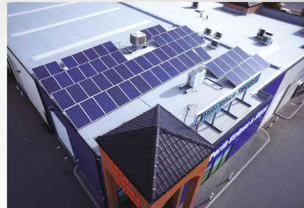
15kw Perth, Australia
